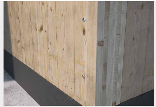
Fastening CLT walls with TBS screws.
