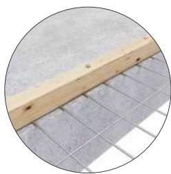
timber batten 40 x 50 mm
