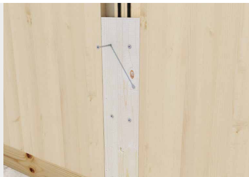
Fastening CLT walls with 0.24 inch (6 mm) diameter HBS screws.
