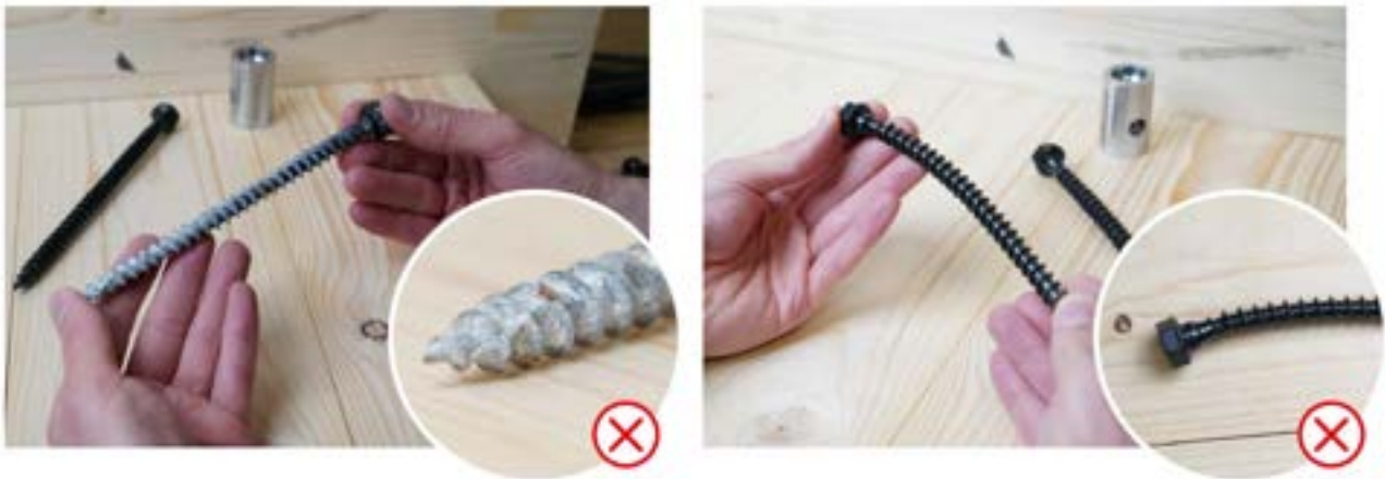
Figure 31. Real examples of visual inspections of used screws. Screw to be discarded due to visible corrosion (left). Screw to be discarded due to visible deformation (right).
