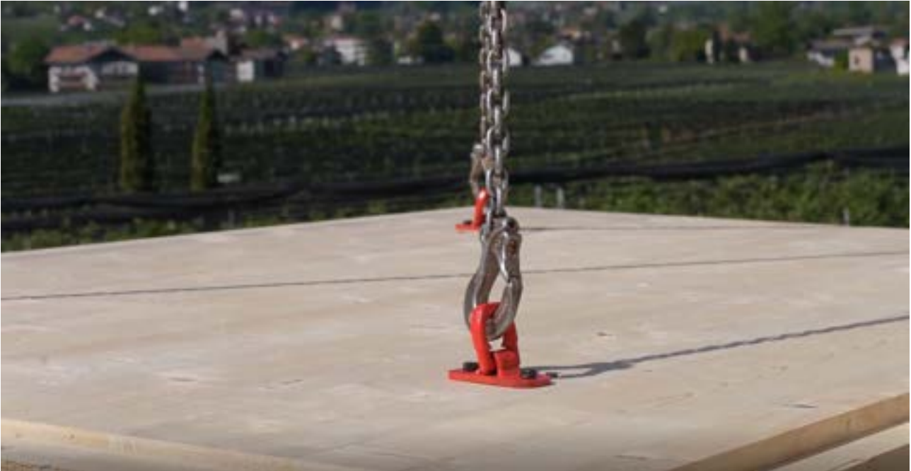
Figure 2. RAPTOR MINI with VGS PLATE on a real CLT-floor-panel lifting application.
