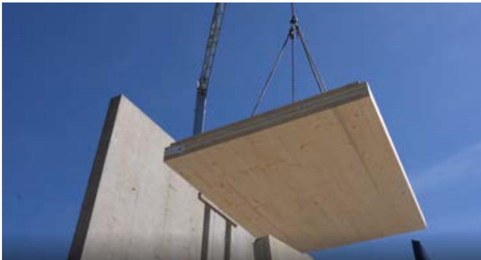
Figure 1. Lifting of a CLT-floor panel on site.
