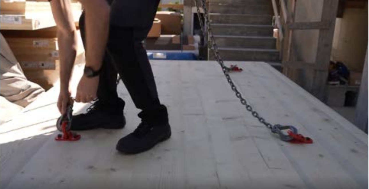
Figure 35. VGS PLATE and RAPTOR MINI in real application conditions.
